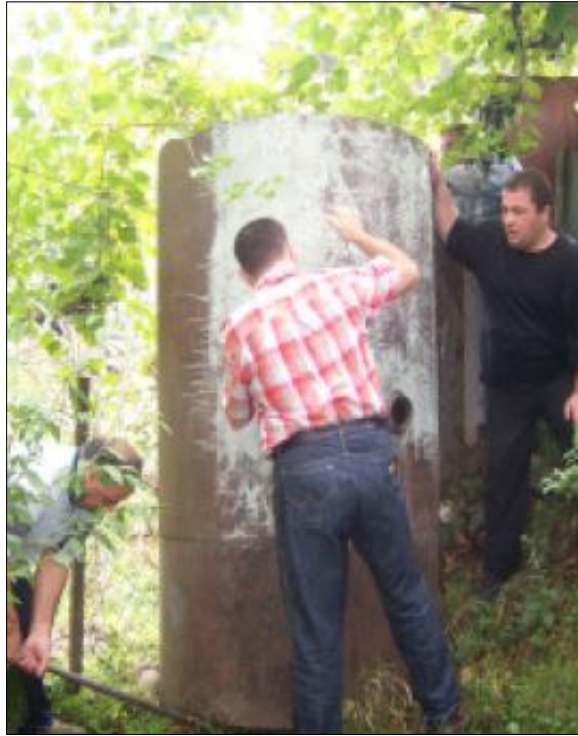
Construction at Gadamshi.
