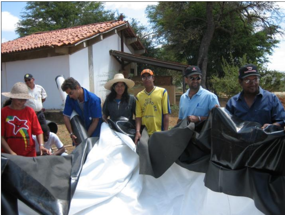
Workers prepared the biodigester for installation.
