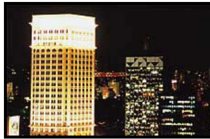
Edificio Plaza Iguatemi, with building climization provided by a natural gas cogeneration system, installed by ABESCO member Union Rhac
