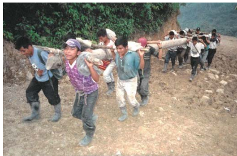
Carrying plant construction materials
