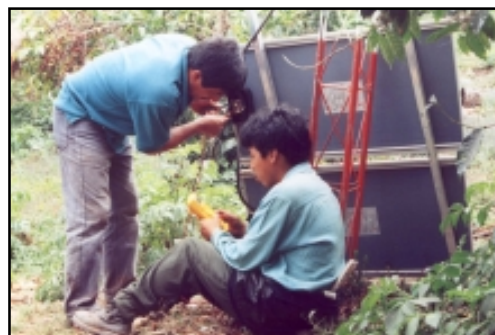
Testing module voltage
