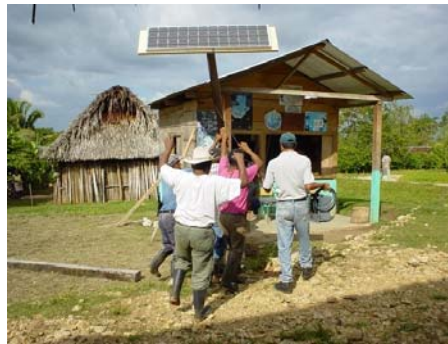
Installing PV for communications and lighting
